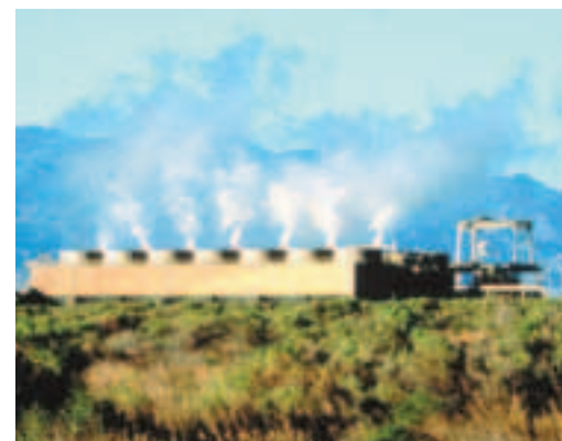
Figure 21 This geothermal power plant in Nevada produces enough electricity to power about 50,000 homes.
